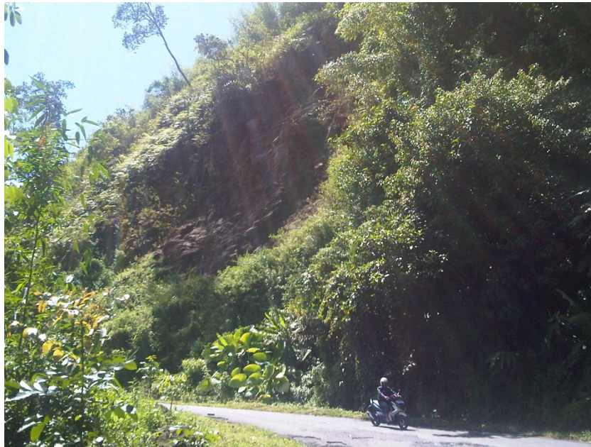
Figure 7. 4 Rockfall at one of road
